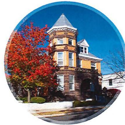
SILVER STREET CAMPUS Historic Jail 312 E. Silver Street
